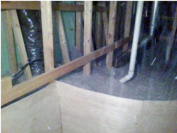
Insulation is blown-in in the area above the furnace room.
