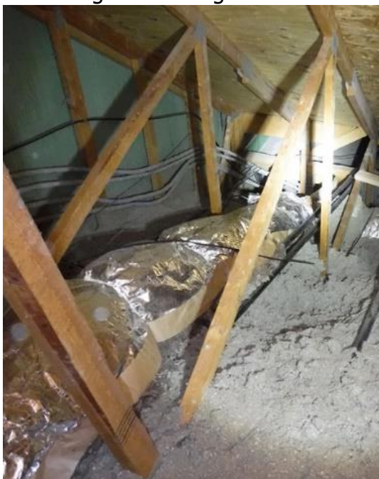
Trunk line insulation position restored and secured with aluminum tape and zip-ties to prevent the insulation from falling off again.
