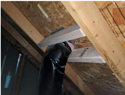
This is the detached bathroom vent and the repair.
